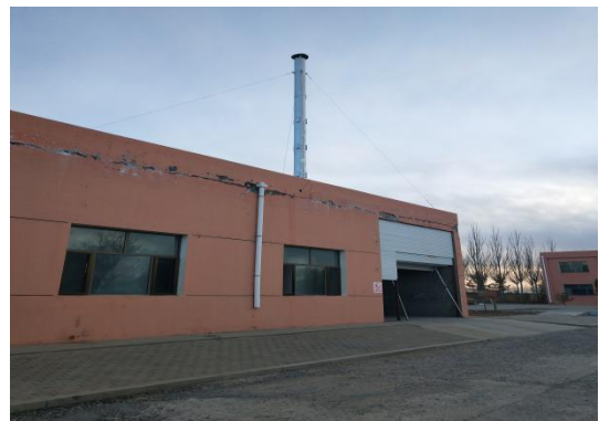
光氧除臭排放口
